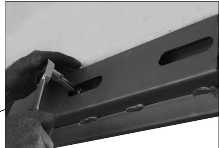
STEP 6: Tighten the coupler anchor bolts.
